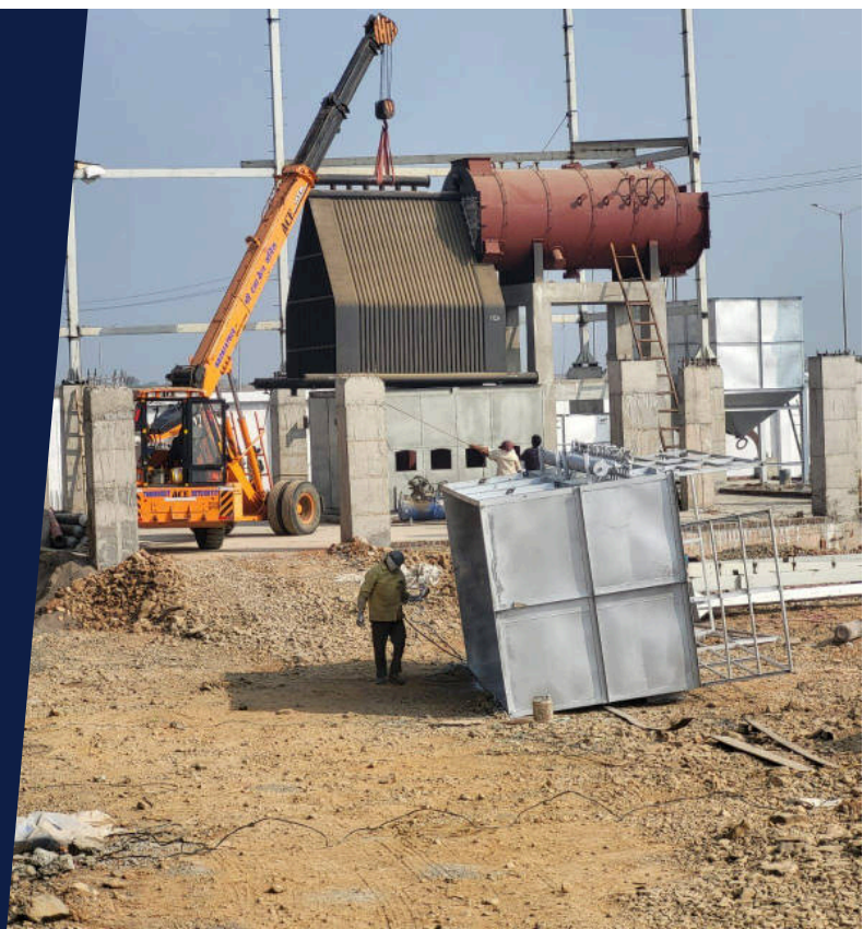
Boiler erection in progress at a client site
